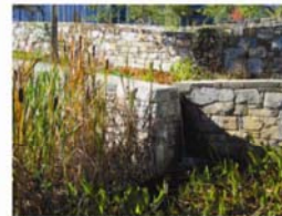
Bio-retention With Retaining Wall
