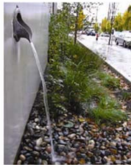
Bio-retention With Retaining Wall
