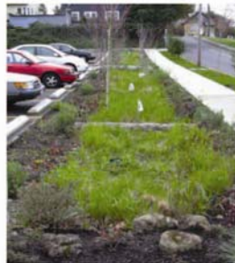
Infiltration Trench for Pavement Runoff
